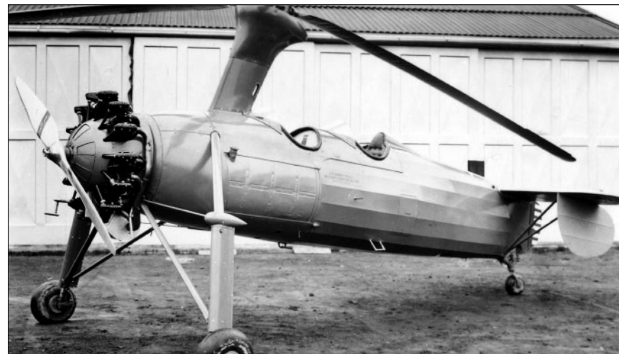
The U.S. Army Air Corps' first helicopter, the Platt-LePage XR-1A (S/N 42-6581), was based on the German Fa 61. While being repaired following a crash at Wright Field, an order for seven YR-1As was canceled. The aircraft was sold to Helicopter Air Transport, which overhauled it and sold it to Frank Piasecki, one of its designers. (Author's Collection)
