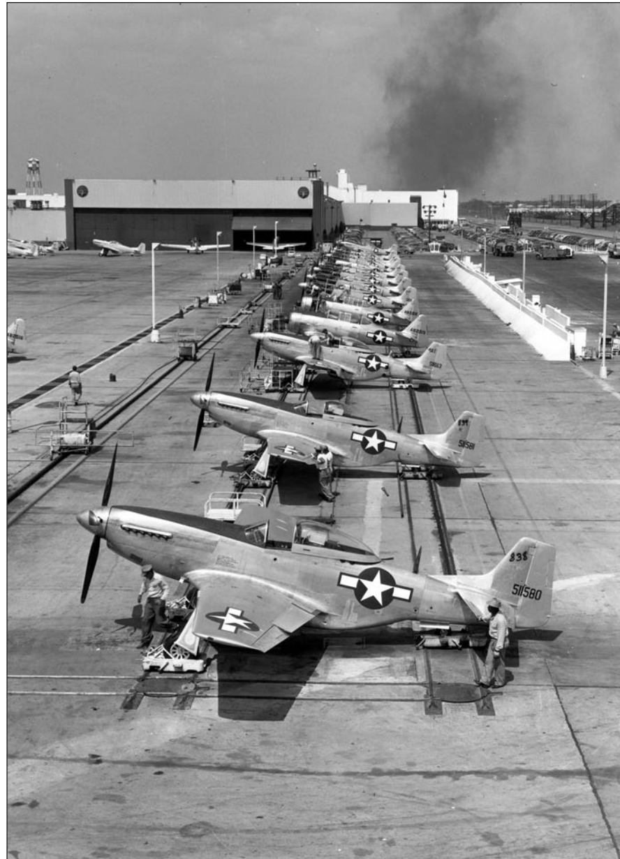
As P-51D/K production ramped up at NAA's Dallas plant, operations were basically similar, but as can be seen in this view of the engine run-up area, AT-6s were mixed into the equation.
