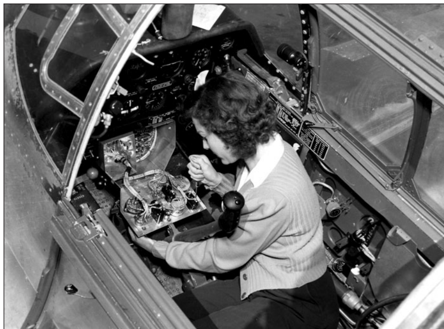
With the wooden pilot's seat removed, a female worker has easier access to cockpit instrument panel wiring although the control stick remains a barrier (aircraft's radio call sign is 36-044). During the early portion of Mustang production, workers usually just wore their normal day clothes.
