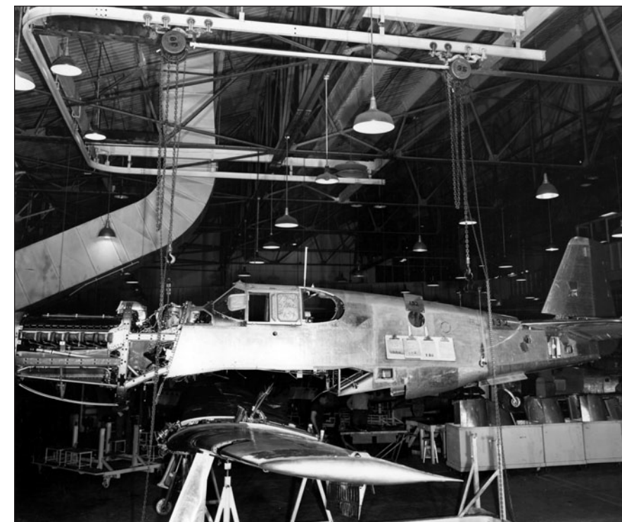
The nearly completed fuselage of P-51A 99-132 is lowered onto its wing. Exact alignment markings on the factory floor allowed precision fitting of the two components.
