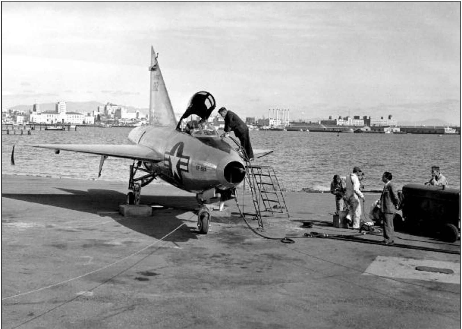
The XF-92A during auxiliary power testing on the shores of San Diego Bay. It was here that Consolidated flying boats made their first flights. The XF-92A, however, would be trucked to the Mojave Desert for its debut. (Convair via Author's collection)
