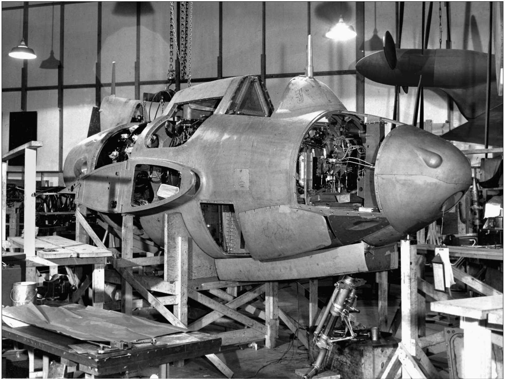
The nacelle (fuselage) of the first XP-56 in final assembly during an engine fit check. The partially open panel above the nose wheel door is the high-lift door that could be deployed by the pilot to reduce diving moments induced by lowering the landing gear and flaps. (Northrop)
