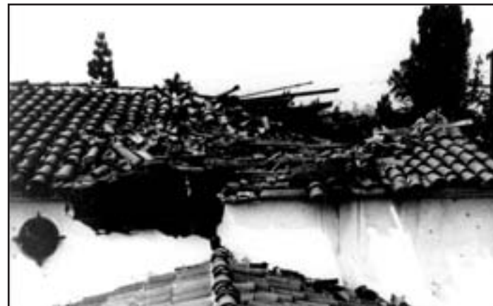
Impact damage at 803 North Linden Drive after the main landing gear of the XF-11 slammed into the Spanish tile roof. (U.S. Air Force)
